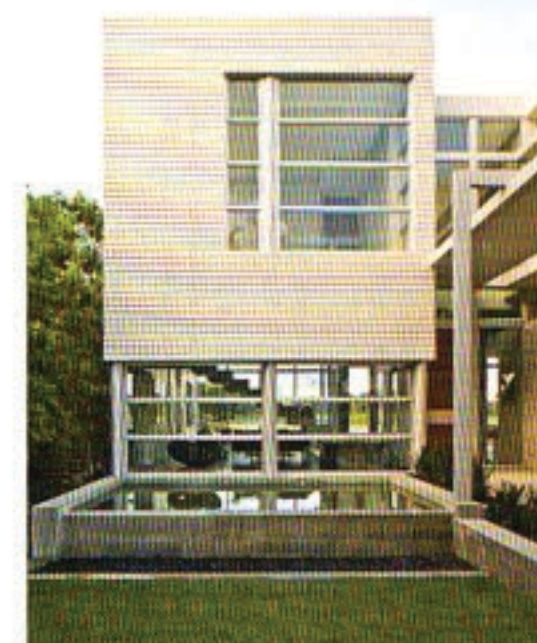
View of the house from the dock, view along the central axis defined on the exterior by a stone wall and view over the lily pond into the great room. All photos by Robin Hill.
